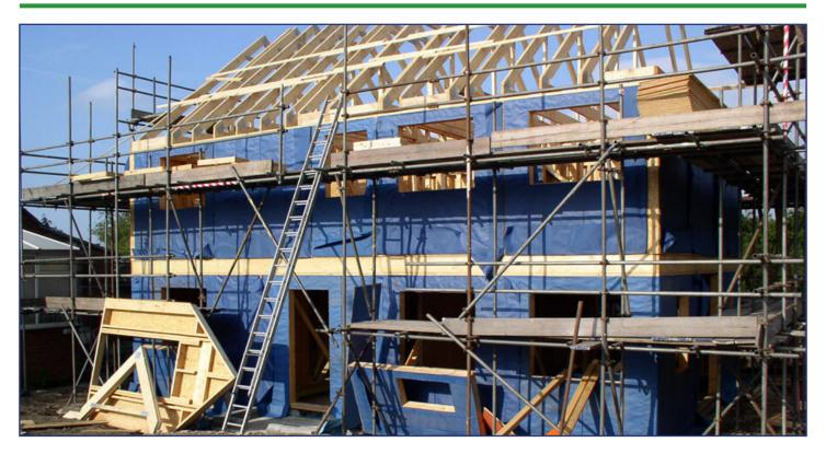
TFS has pioneered the development of patent protected pre-bonded breather membrane panels, in response to increased demand for timber framed construction. This innovative design ensures that application of the breather membrane does not affect the breathability of the panel. It is water resistant but air permeable and is located on the cold side of an insulated wall.
