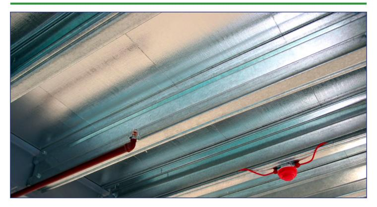
Class o foil products deliver a major contribution towards fire safety in commercial and residential buildings. TFS offer fire retardant foils that are factory bonded to a range of substrates to achieve BS 476 Class o certification, including particleboard, plywood and MDF.
